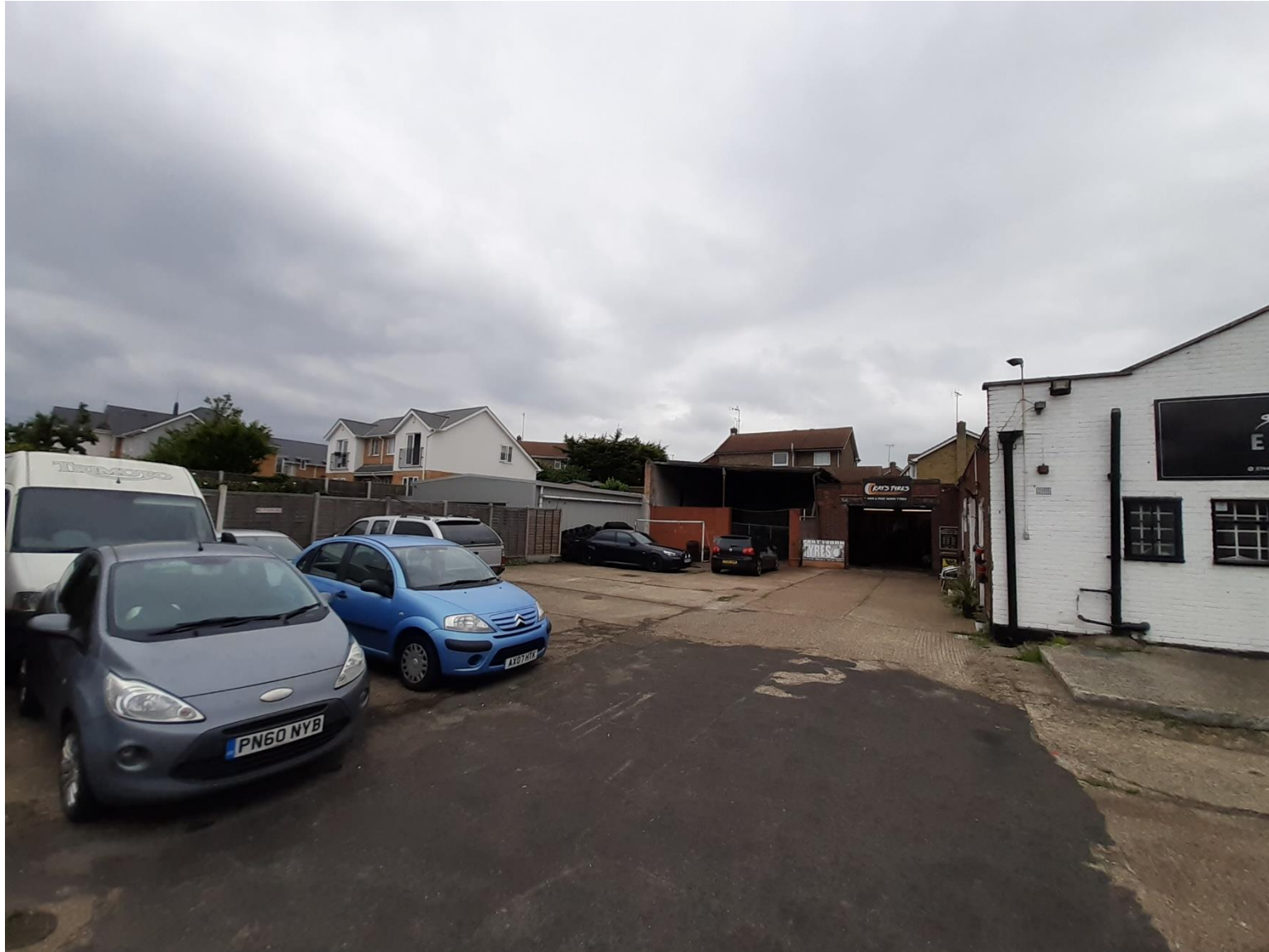
The front elevation of the building on site
