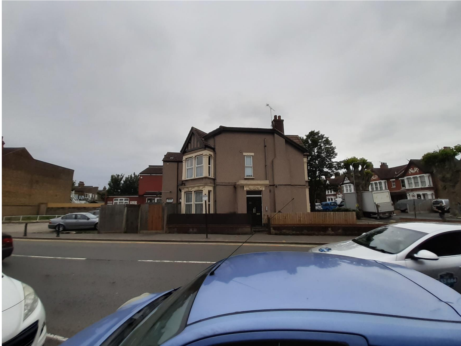
The neighbouring property to the north-west of the site
