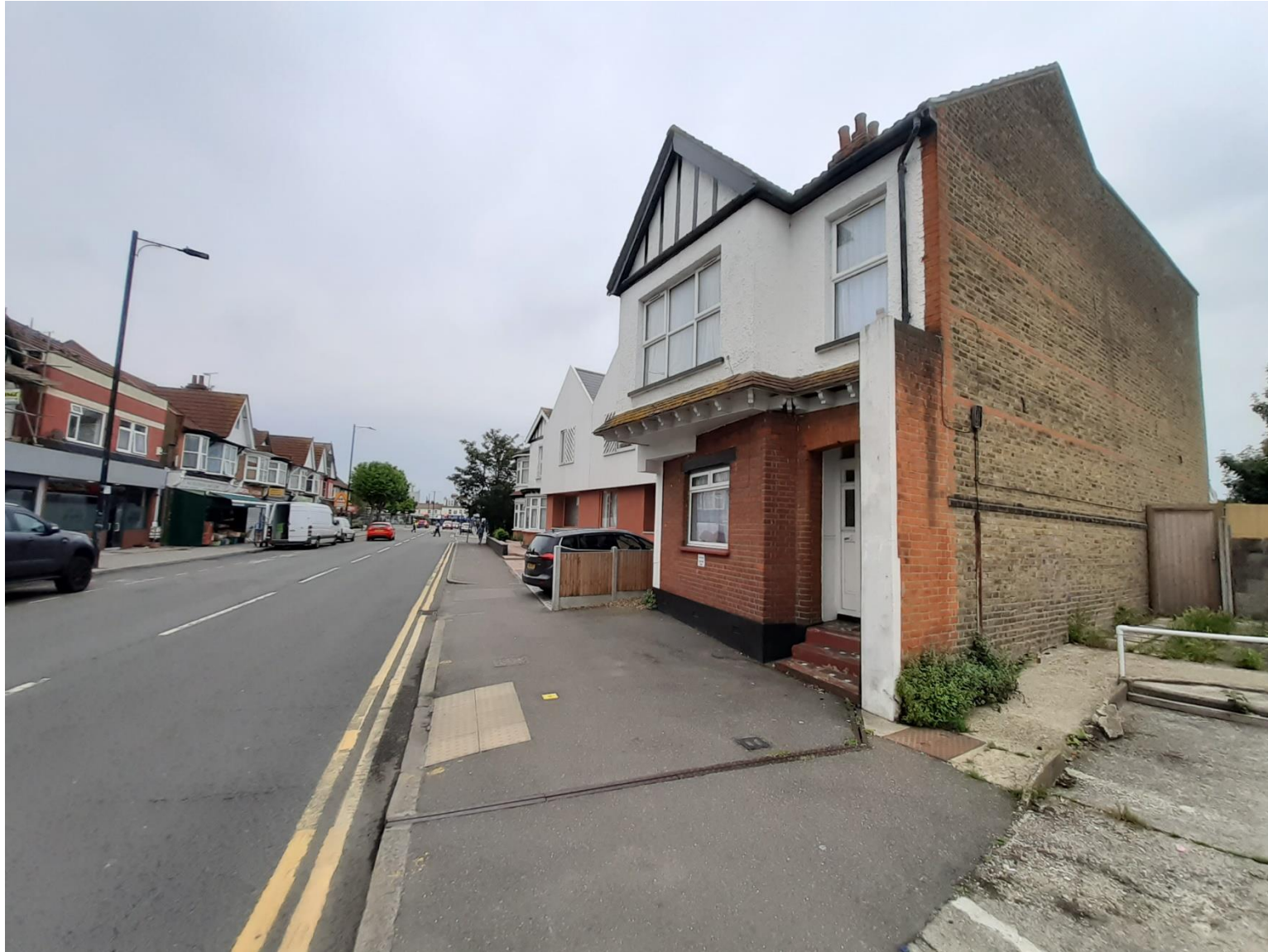
Eastward view on London Road
